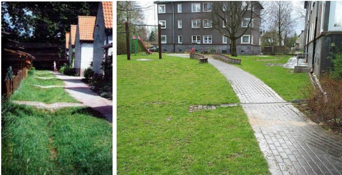
Figure 4: Swale trench system in Gelsenkirchen (left), disconnection in Bottrop (right)
