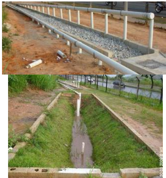
Figure 2. Infiltration trench (left); Detention trench (right)
