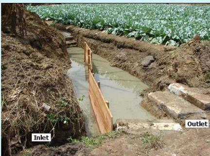
Figure 2: Interconnected pond with hardwood baffles.
