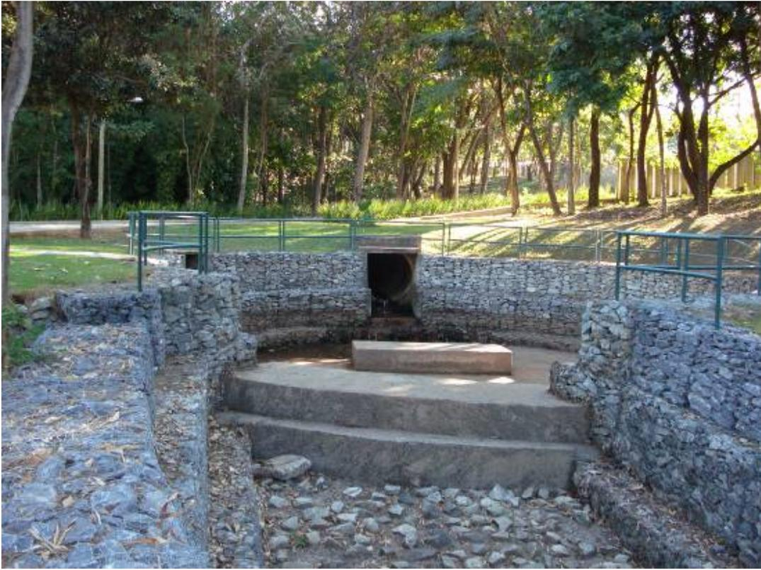
Photo 3: existing gabion and concrete structures in the Lagoa do Nado Park
