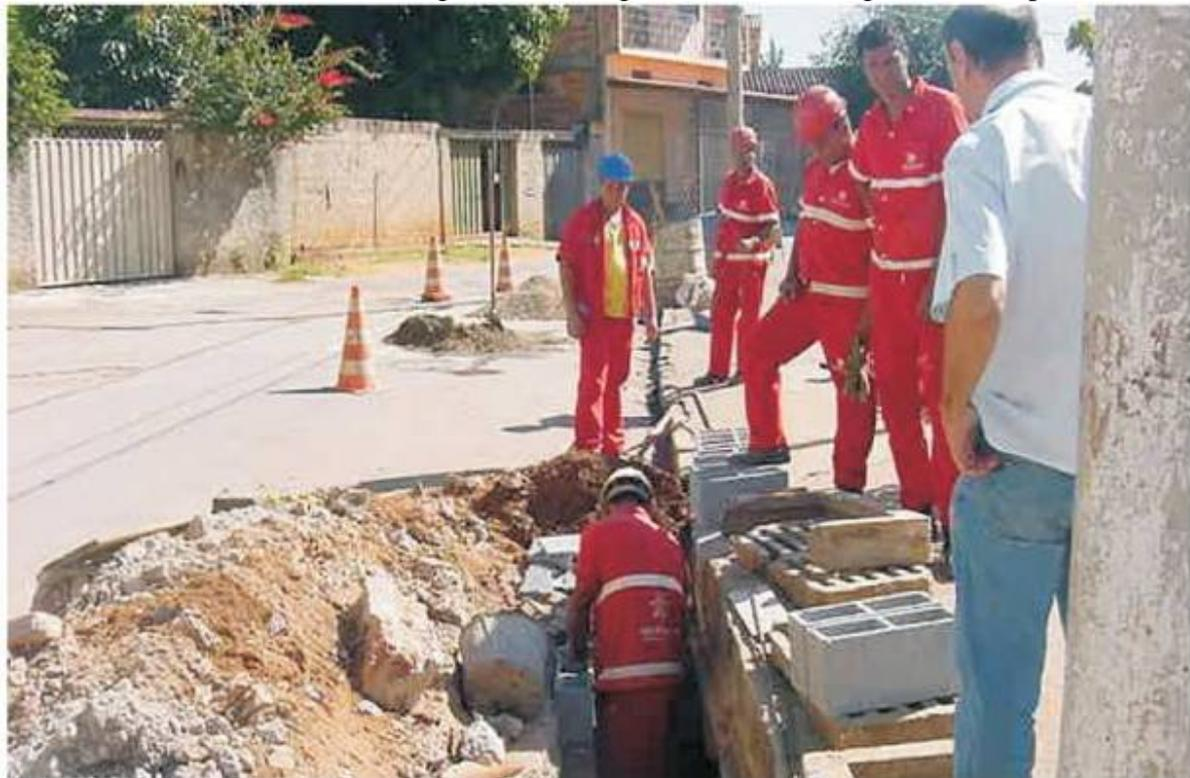
Photo 8: installing gully with permeable bottom, at Vila Guaratã
